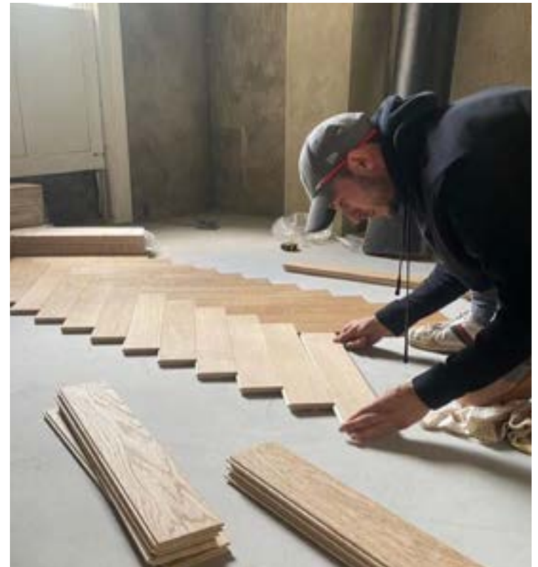
When the compound is dry the floor can be fitted
