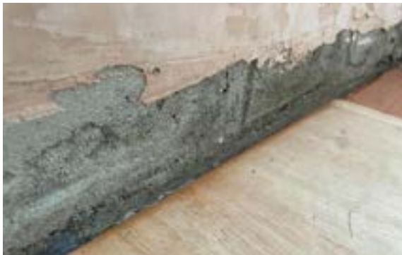
Use silicone in the gaps to avoid leaking
