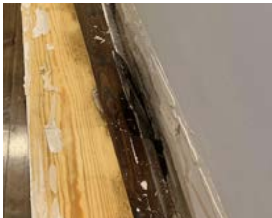
In this property the skirting was removed
