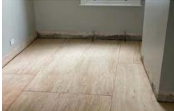
Use ply across the entire area...
