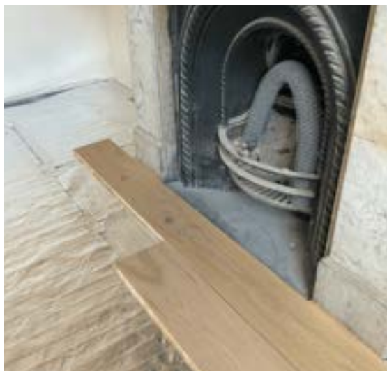
Float wood floors directly onto foil, electric underfloor heating system
